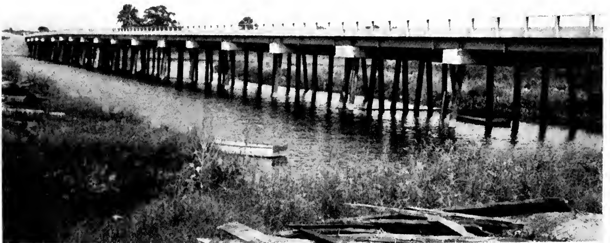
NEW TUCKAHOE CREEK BRIDGE BETWEEN CAROLINE AND TALBOT COUNTIES
